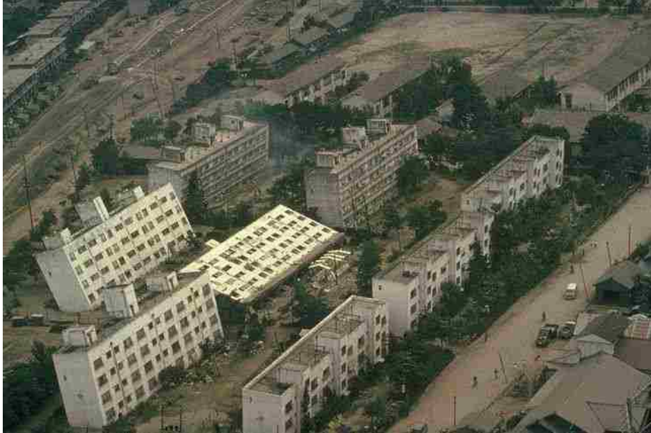
Figure 2.1. Bearing capacity failure of the Kawagishi-cho apartment buildings due to flow liquefaction (USGS).
